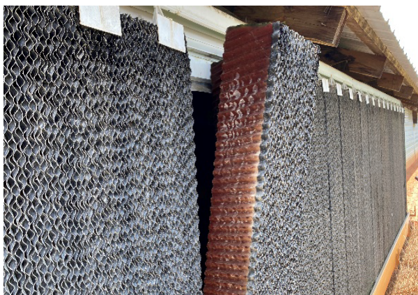
Figure 7. Pad surface is dry, interior is still wet
