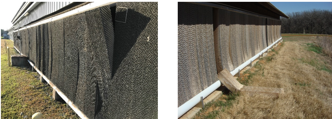
Figure 11. Pads losing rigidity due to high Ph water
