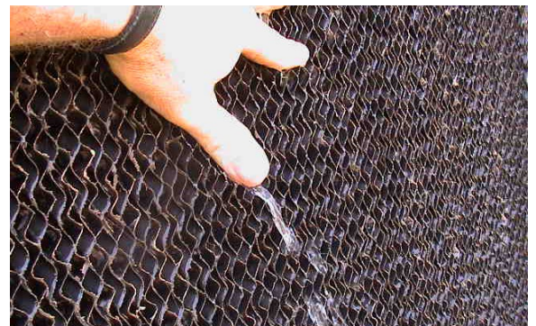
Figure 6. Checking for water flow over pad surface
