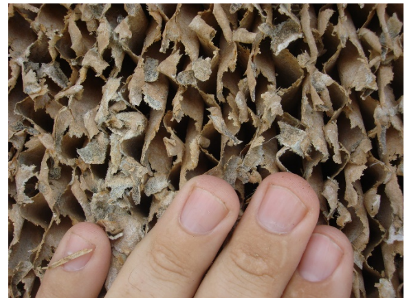
Figure 4. Softened pad surface
