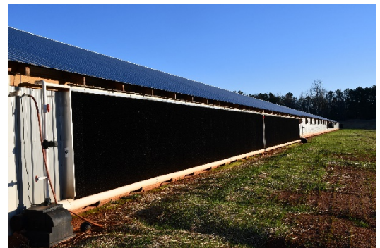
Figure 1. Barn equipped with evaporative cooling pads
