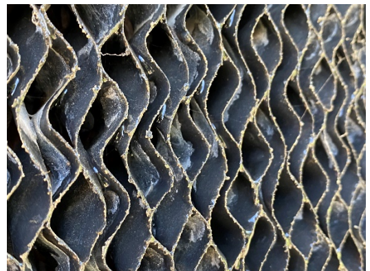
Figure 2. Water flowing over surface of Evaporative Cooling Pad
