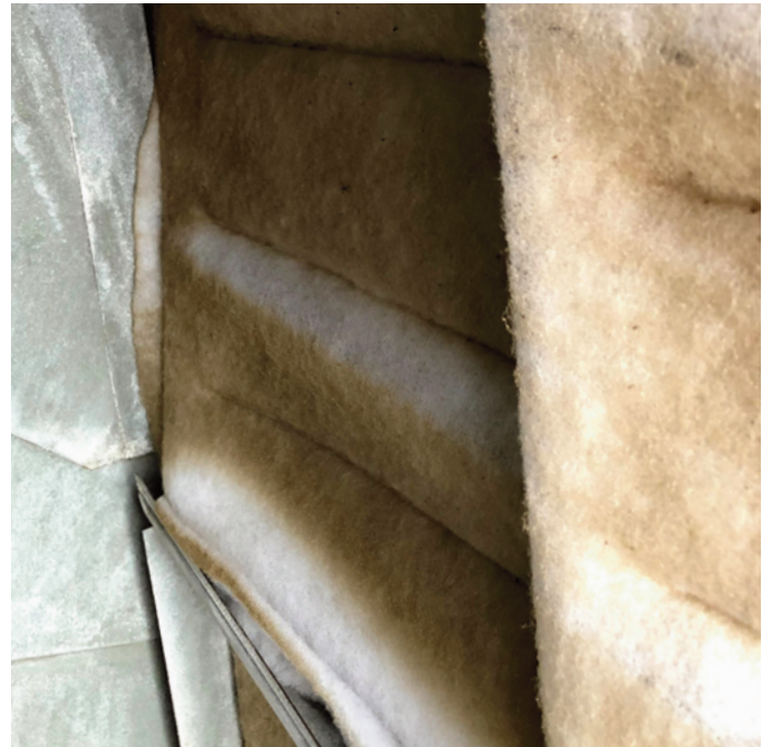
Figure 76. Dirty air filters
